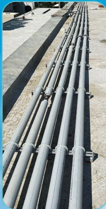
LIP Channel Hanging System at Site
